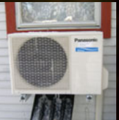
Freezing Resistance and Field Tests Field tests are conducted under actual conditions of use in the middle of winter.
